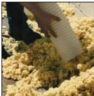
Insulation Removal
