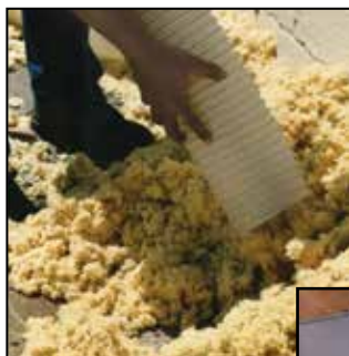
Insulation Removal
